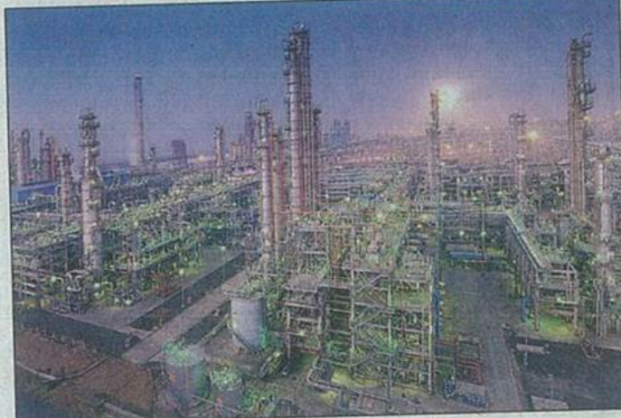
The OPaL plant located at Dahej
